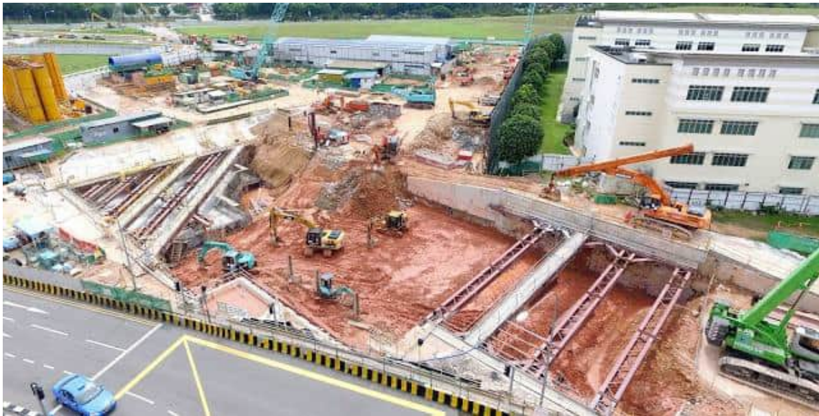
Figure 3-23 Example of Bottom-Up Construction at Woodlands South Worksite [W-7]
