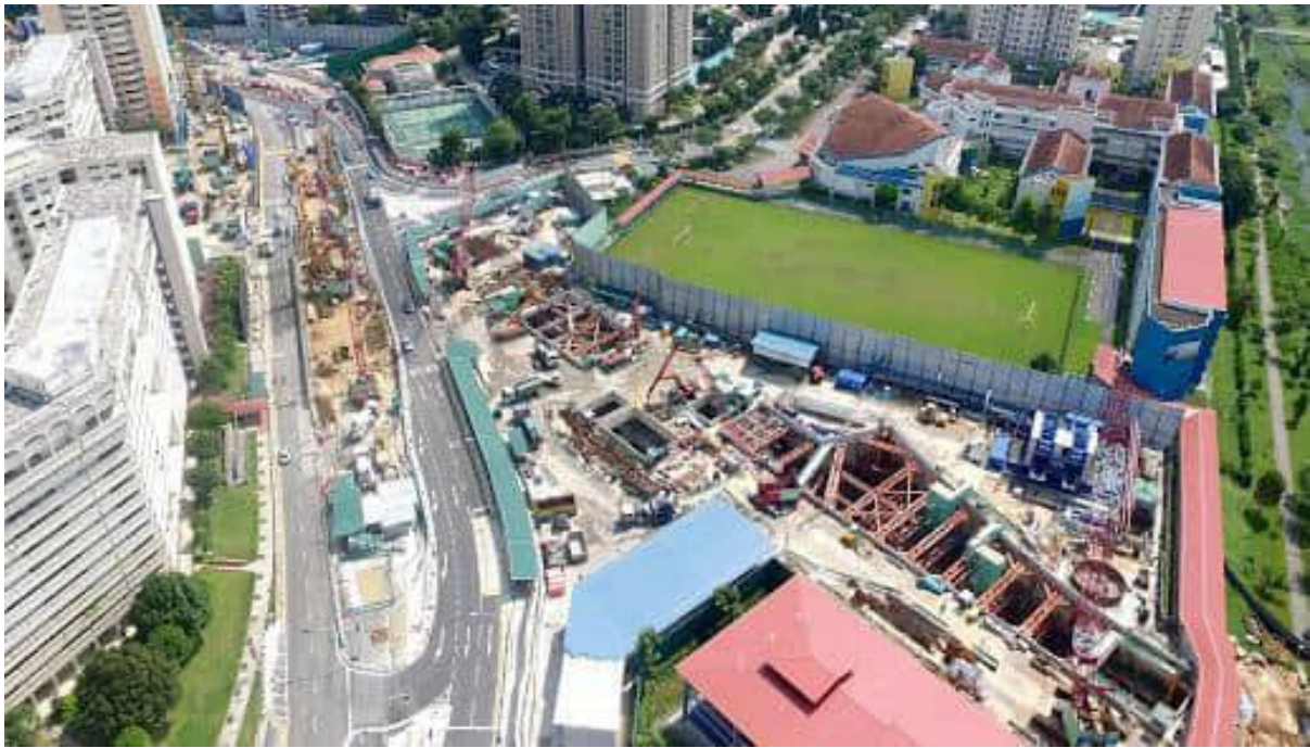
Figure 3-11 Example of Road Diversion and Traffic Realignment at Sin Ming Avenue End April 2016 [W-3]
