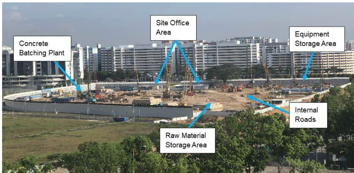
Figure 3-14 Example of a Typical Worksite Layout [O-6]
