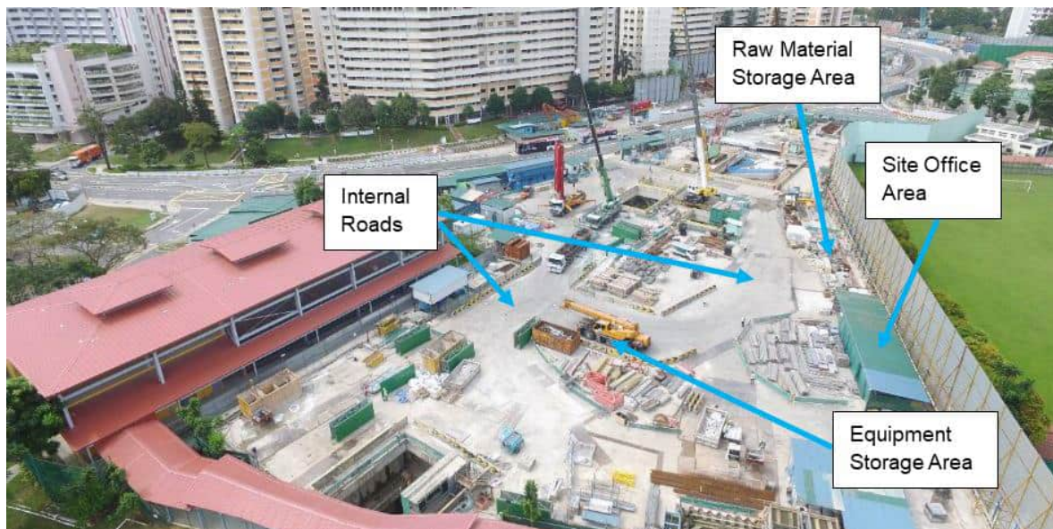
Figure 3-15 Bright Hill MRT – Example of a Temporary Worksite Area [W-5]
