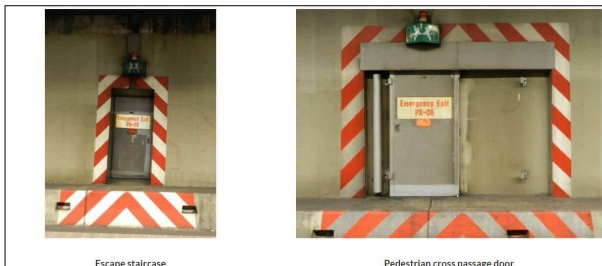
Figure 3-28 Example of Escape Staircase and Cross Passage Door [W-92]
