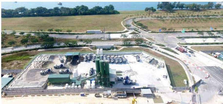
Figure 3-30 Example of a Batching Plant at Marina South for Tunnel and Station Box Construction [W-8]
