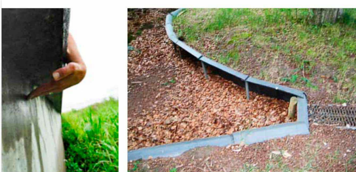
➤ Fencing design options. (Left) On US Highway 441, Florida, a concrete barrier wall with lip limits access to roadways. (Right) Metal flashing is designed to funnel animals, especially reptiles and amphibians, to a highway crossing grate (photos by Marcel Huijser).
