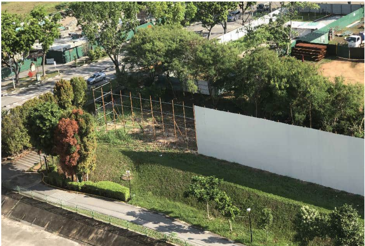
Figure 3-8 Examples of Site Hoarding Erection [O-6]
