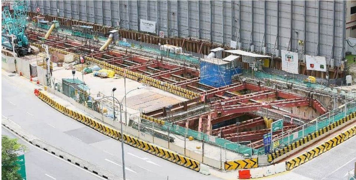
Figure 3-22 Examples of Top Down Construction at Lentor MRT Worksite [W-22]
