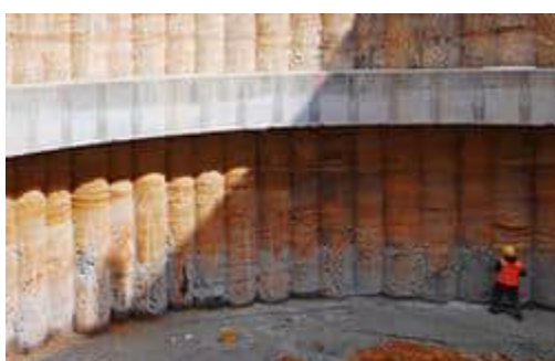
Figure 3-12 Examples of Secant Bored Piles [W-81]
