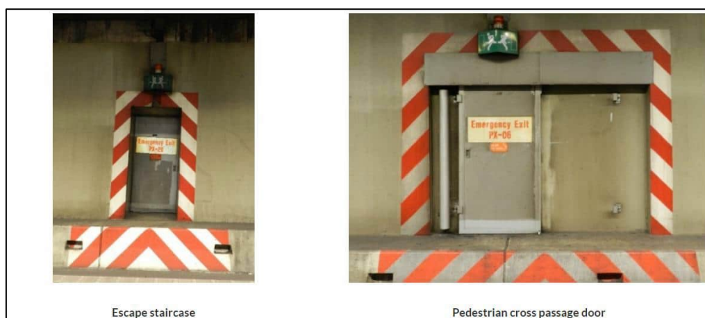
Figure 3-29 Examples of Escape Staircase and Cross Passage Door [W-94]
