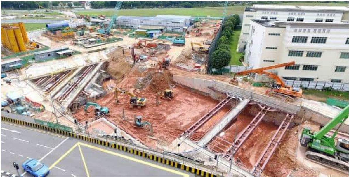
Figure 3-24 Examples of Bottom Up Construction at Woodlands South Worksite [W-7]
