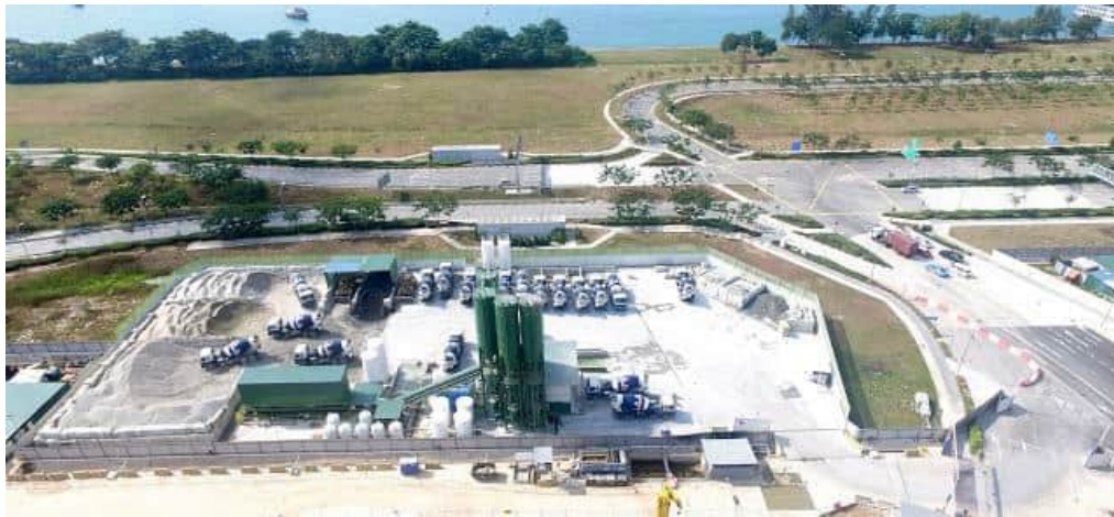
Figure 3-32 Examples of Batching Plant at Marina South for Tunnel and Station Box Construction [W-8]
