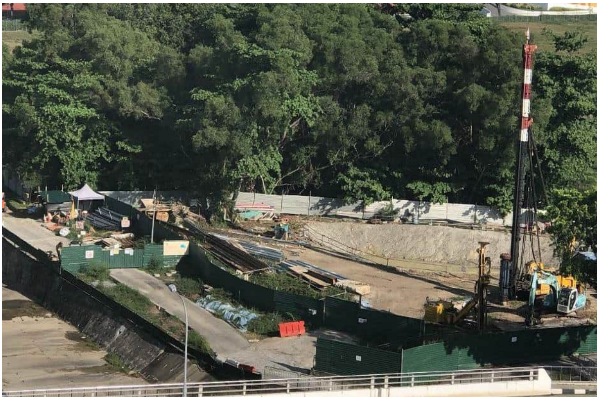
Figure 3-10 Examples of Slope Cutting Works [O-6]
