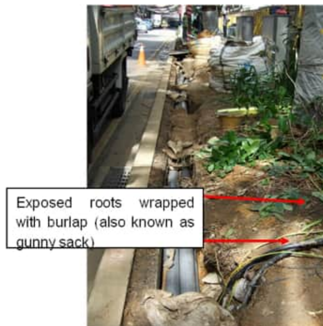
Figure 9: Tunneling under roots.
