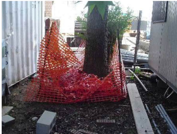
Figure 7: Inappropriate installation/maintenance of TPZ during construction.
