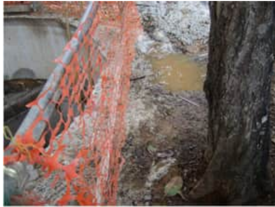
Figure 5: Construction cement deposited at tree base.
