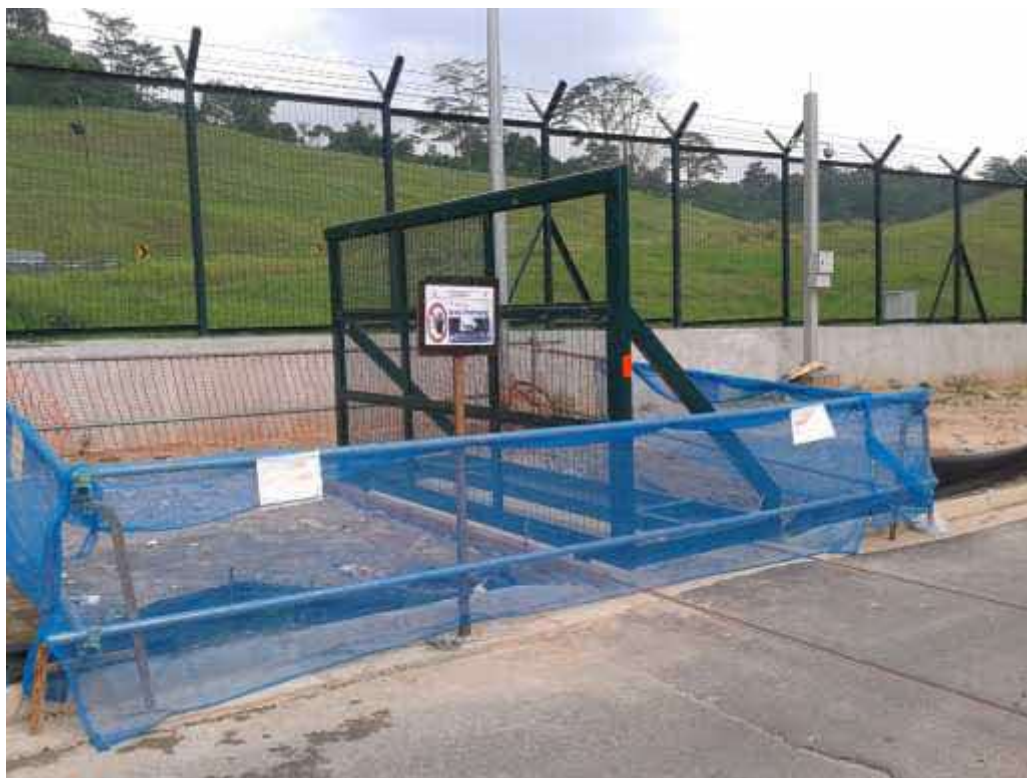
Cordon off work zone around gate installation
