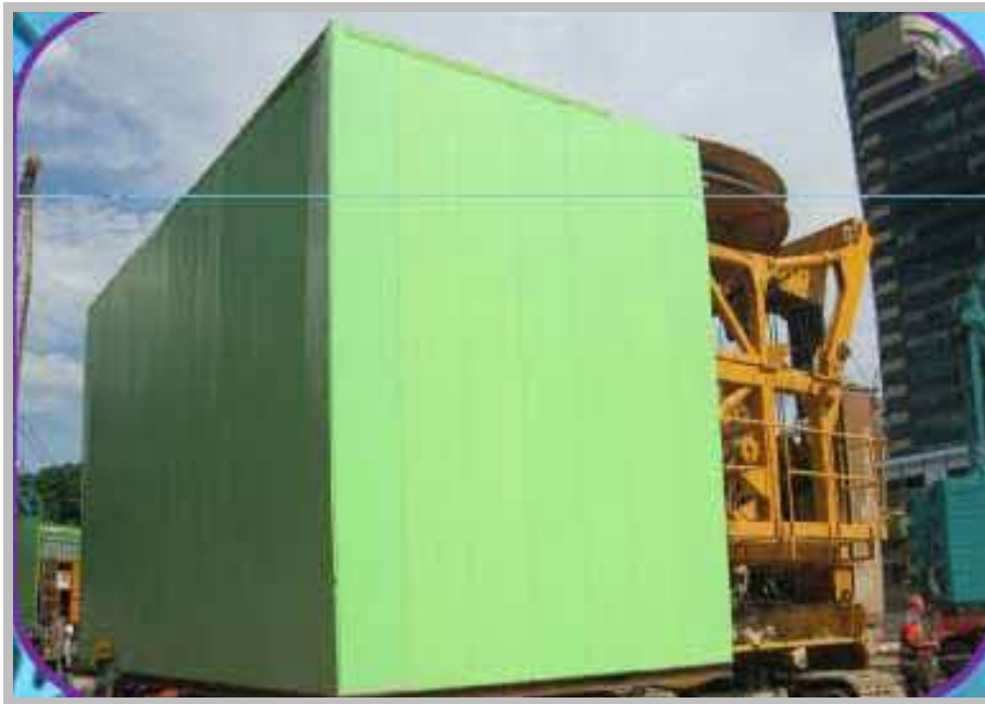
Noise enclosure on D-wall cutter machine
