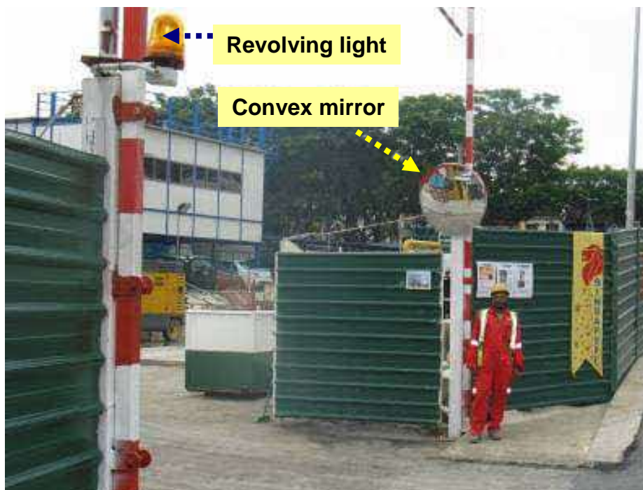
Site entrance equipped with revolving light and convex mirror to enhance pedestrian safety. Full-time banksman deployed to guide vehicles exiting the worksite
