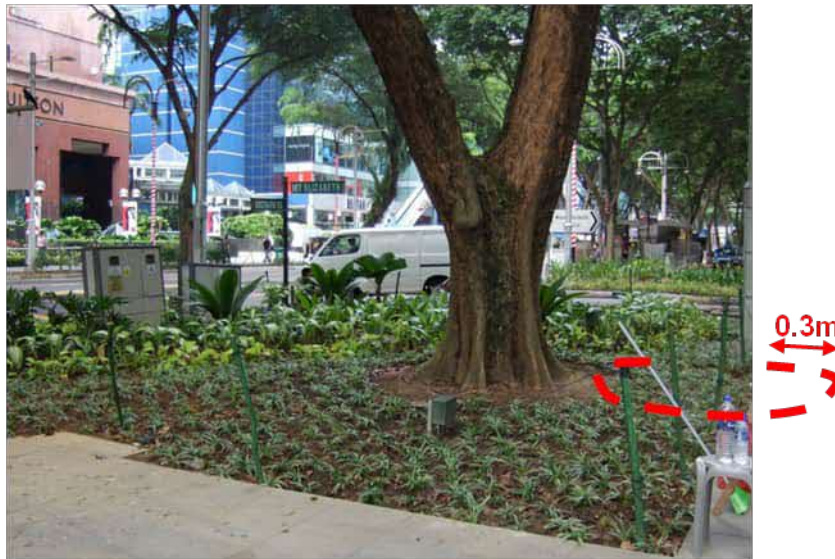
Figure 10: New plantings at a minimum distance of 300mm (all round) from root collar
