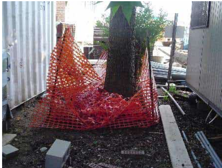
Figure 7: Inappropriate installation/maintenance of TPZ during construction.
