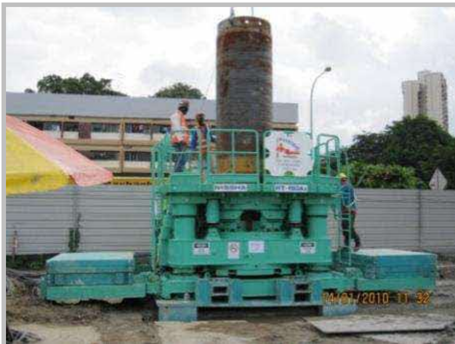
Use of silent-piling machine (for suitable soil conditions)
