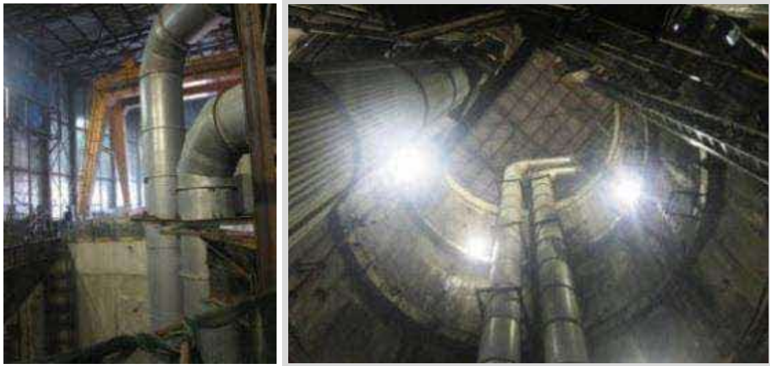
Full acoustic enclosures designed with air ventilation system and adequate space for plants and machineries to manoeuvre
