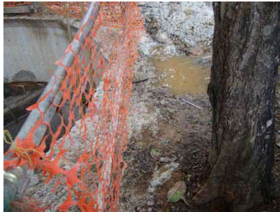
Figure 5: Construction cement deposited at tree base.
