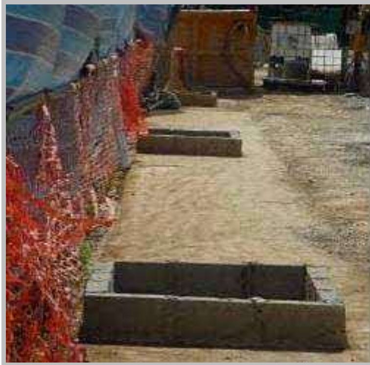
Use of bund wall to protect silty runoff from entering the public drain
