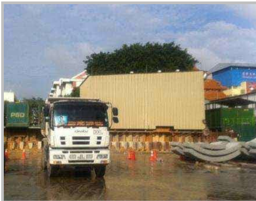
Large acoustic enclosures on slurry treatment plants
