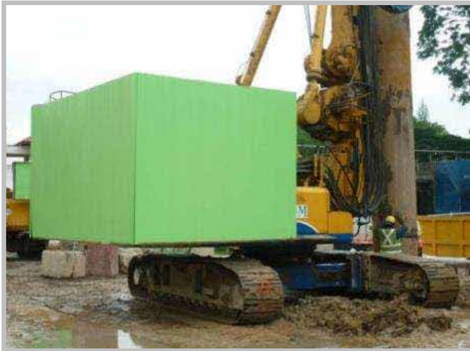
Noise enclosure on boring rigs
