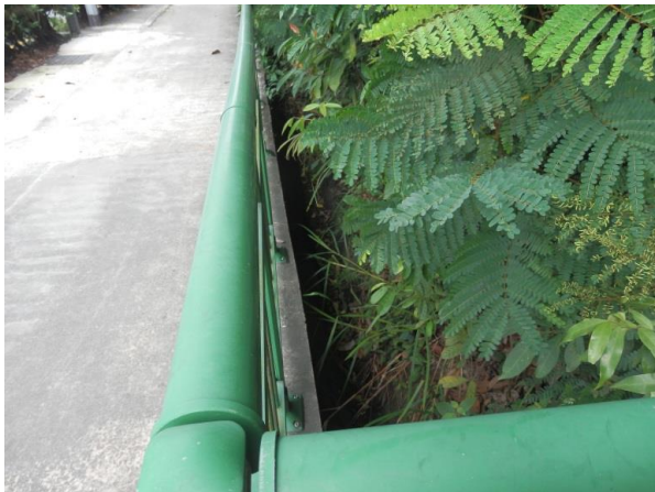
Stormwater drainage channel between the pavement and CCNR forest. (ERM 17.06.15)
