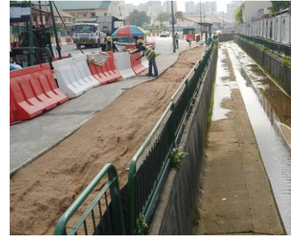
ECB positioned between the surface waterbody and Thomson Line construction activities (ERM, 12.11.2015)
