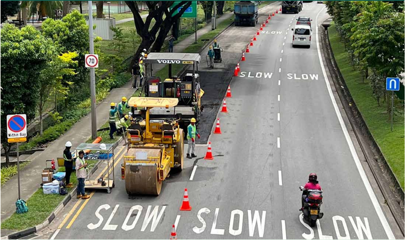
Plastic pavement mixes being field-tested along West Coast Highway
