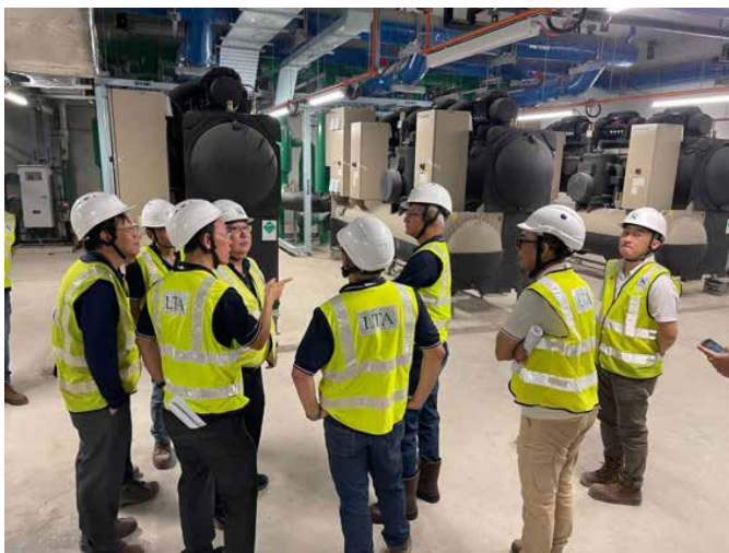
Safety and progress review at Marine Parade Station on TEL Stage 4
