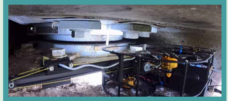
Viaduct bearing inspection using drone and AI
