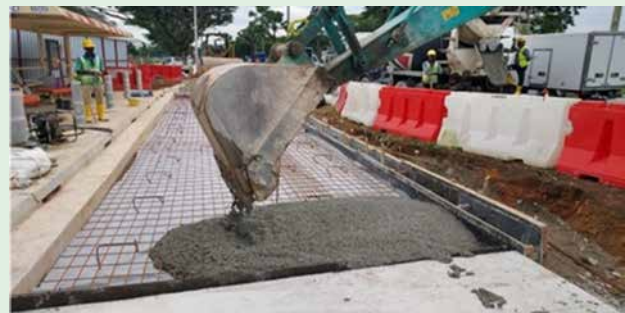
Trial cast of a reinforced concrete bus bay using low-carbon concrete
