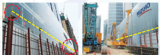
Figure 6: Photo-electric beam sensors and visual indicators
