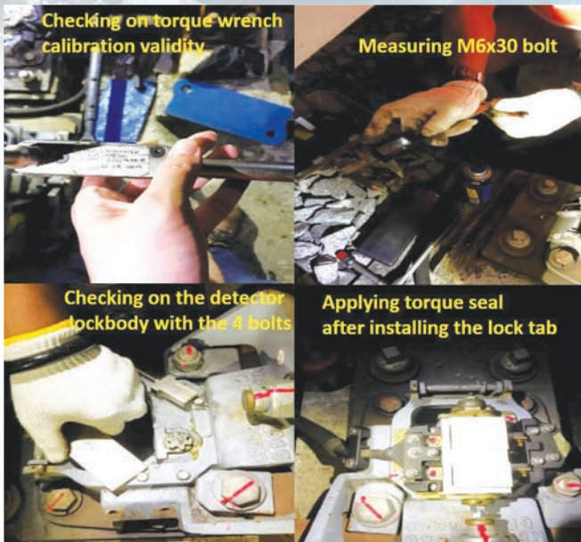
Figure 3: Point Machine Condition Inspection
