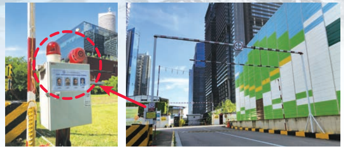
Figure 3: Customised Height Limit Alarm Warning System
