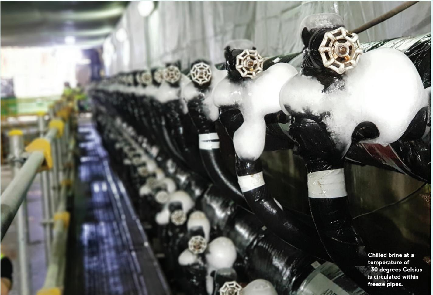
An engineering feat is taking place 40 metres under Marina Bay Station, where giant ice walls are helping engineers to safely excavate tunnels for the Thomson-East Coast Line (TEL). Find out how this cool technology works.
