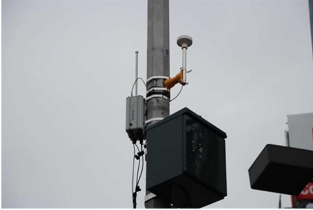
Dedicated Short Range Communications (DSRC) Beacons which will be installed in due course
