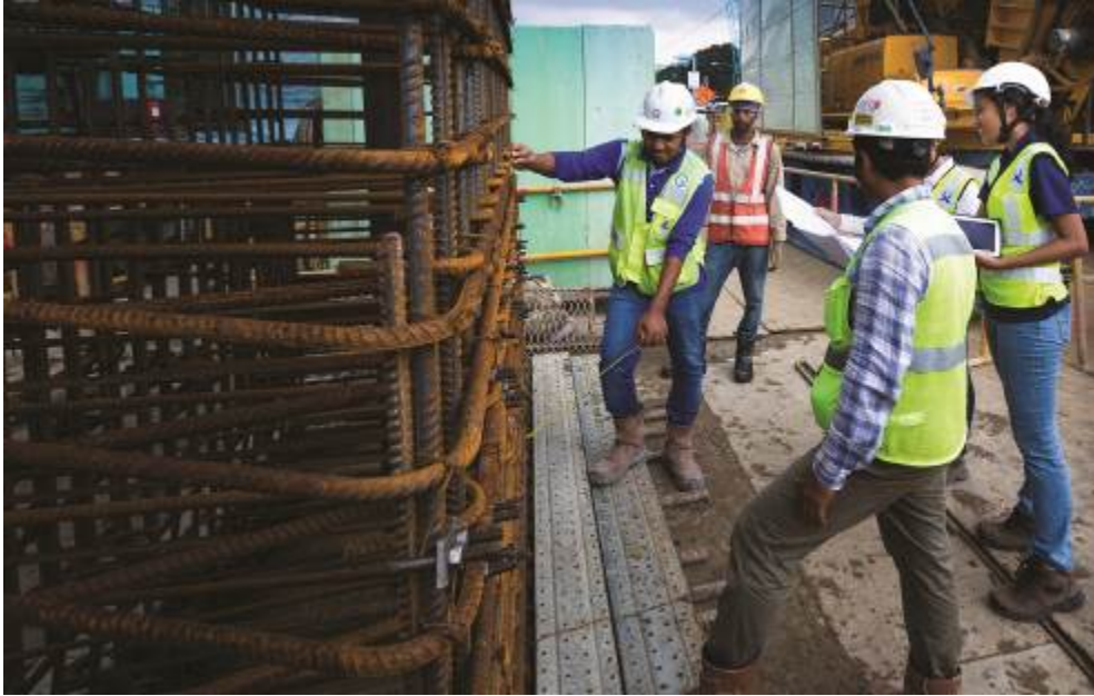
Lowering of Rebar Cage of Diaphragm Wall by Jason Goh
