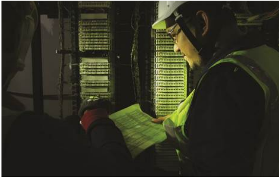
Wiring Verification by June Yeo
